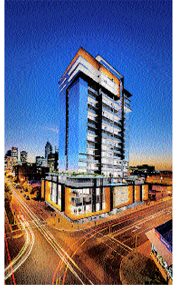
Construction work has started on Blackburne's Oracle apartments.
